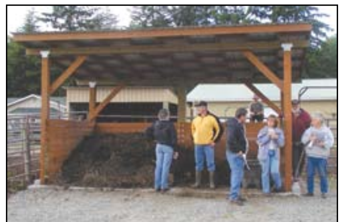
Covered horse manure storage/composting facility.
