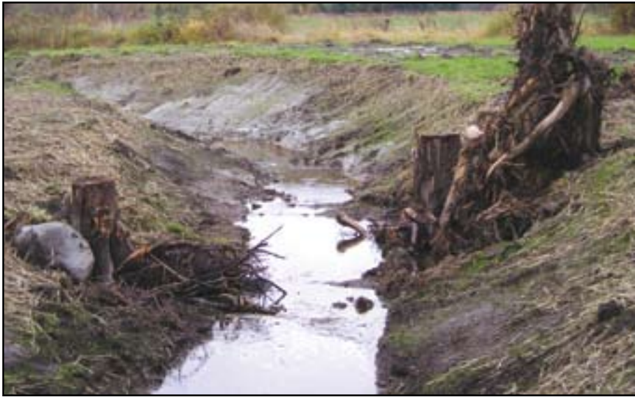
A new channel improves spring-fed water flow into Campbell Creek, enhancing Coho spawning and rearing habitat.
