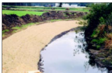
Notice how much wider the stream channel appears in this photo than in the prerestoration photo to the left. Dredge spoils are stacked in the field and the banks are lined with straw mats to prevent erosion.
