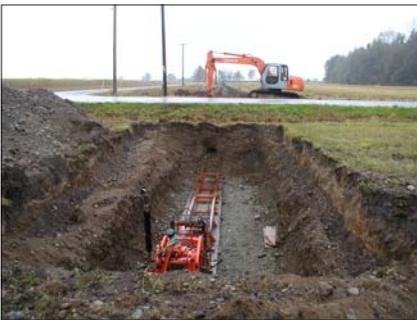
Manure pipeline installation under a road. Pipelines lower the cost of applying manure to distant fields.
