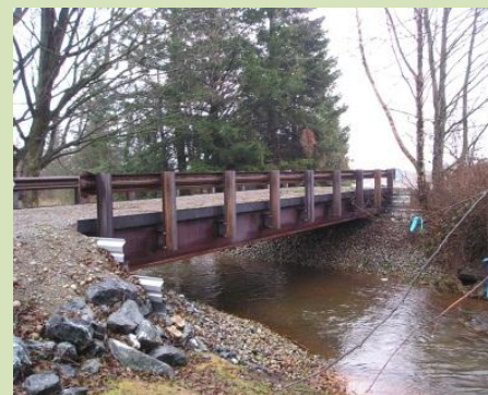
After: Bridge crossing on blueberry farm was installed in September 2013 by the Nooksack Salmon Enhancement Association & Harkness Construction.
